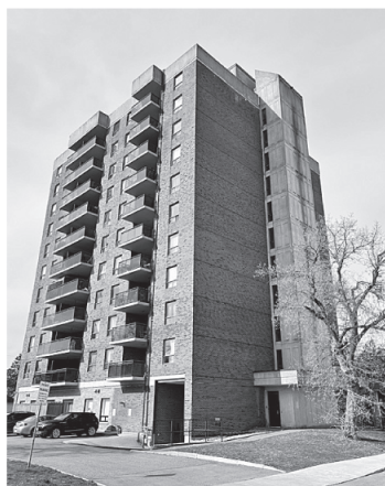
1144 Rockingham Avenue with its striking monolithic stair towers.
