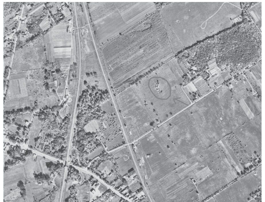
A 1938 air photo of Billings Bridge and Applewood Acres with possible future Crocus Avenue elm trees circled. Credit: uOttawa NAPL Index A6352
