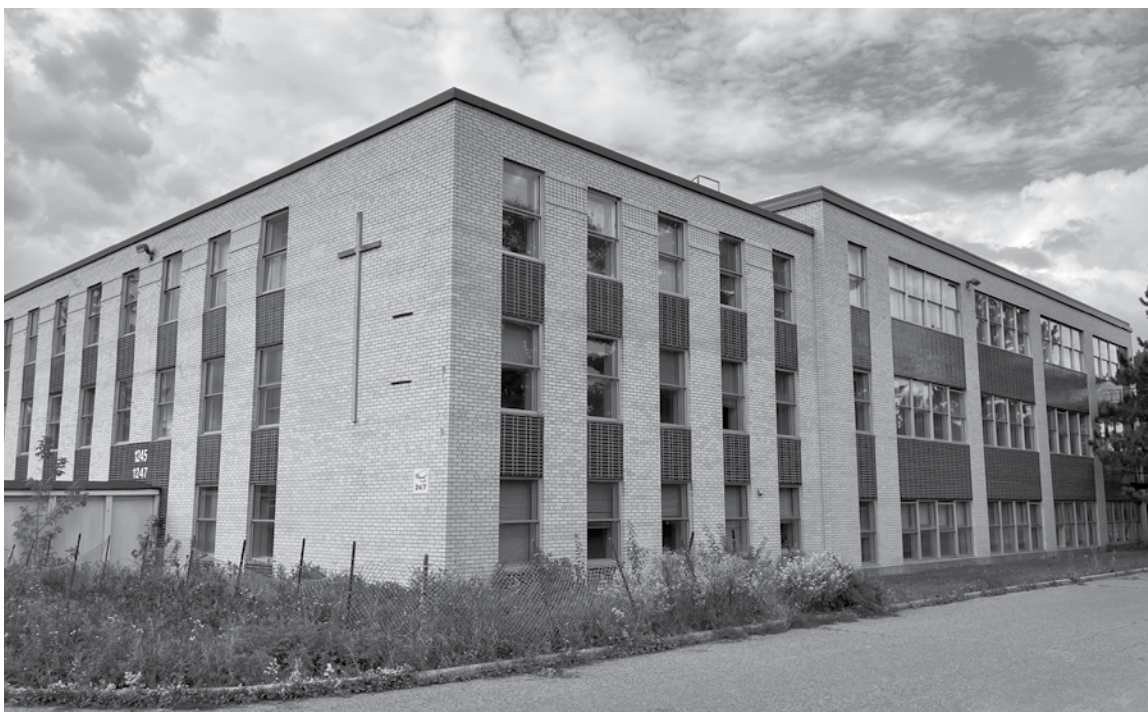
Education wing on the east side of the former Diocesan Centre; photo credit: Chris Weibe
