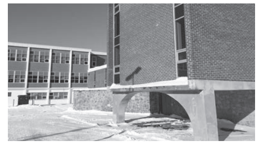
Textured wall treatments at the rear of the building
